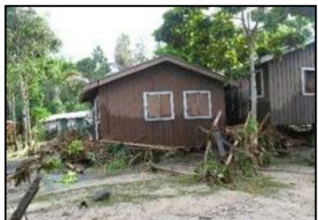
Homes Destroyed by Tropical Cyclones in Fiji
